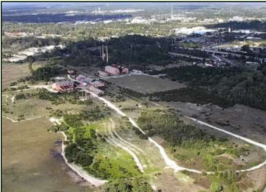
Aerial view of the LCP Chemicals site prior to demolition of the buildings. Photo by Daniel Parshley
