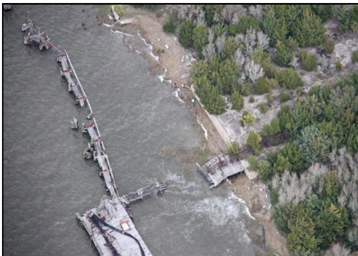
Salt dock located on-site
