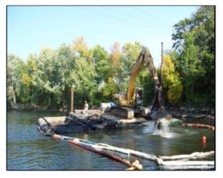
Capping – Cover the contaminated sediment with layers of sand, silt, gravel and rock designed to contain and isolate the contamination. This is also called "containment."
